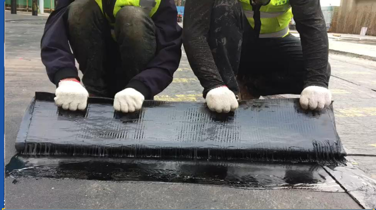
⑦ Brush Coating and Pave membrane
