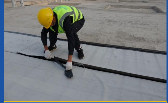
③ Remove Overlap Isolated Tape
