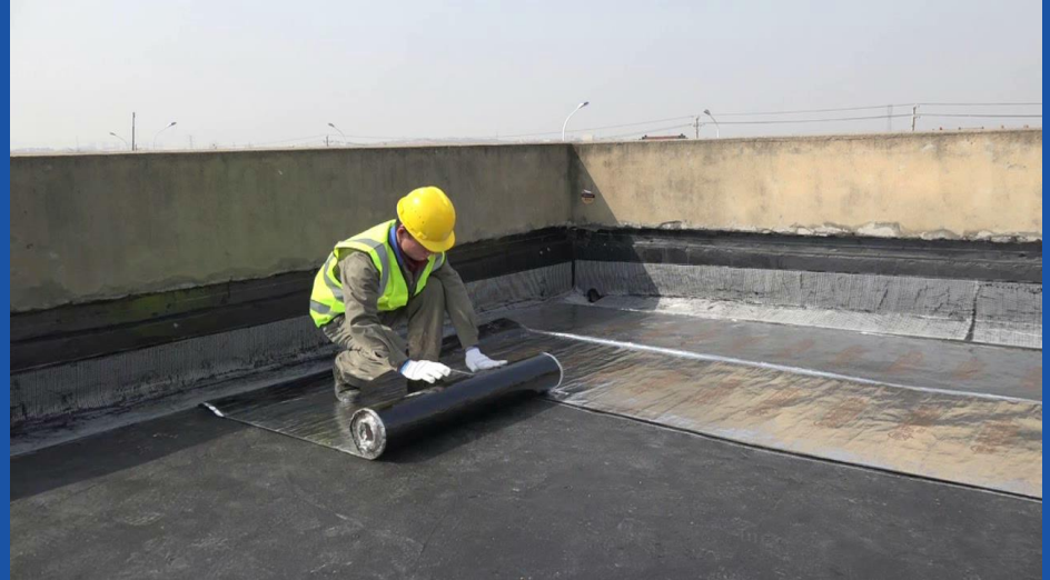
Avoid Edge Warping, the membrane curling
