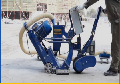
① Substrate Shot-blasting Treatment
