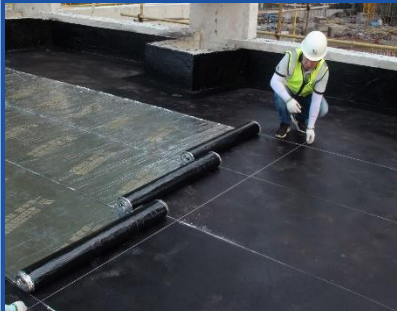
⑤ Positioning and lining
